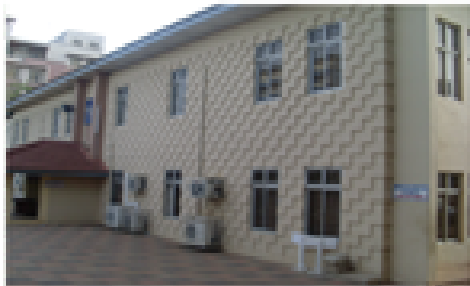
MDC Old Renovated Block
