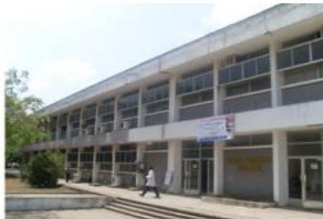
First Medical School Building (Basics Sciences Building)
